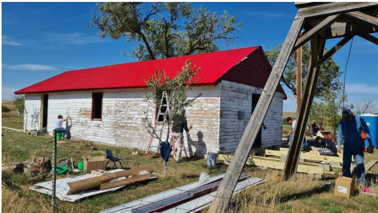
Figure 13. New roof, new paint, new porch!
